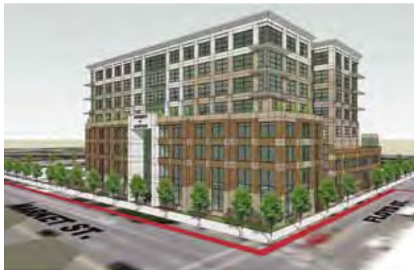
The Foundation broke ground on the eight-story, 160,000-square-foot Nucleus building.
